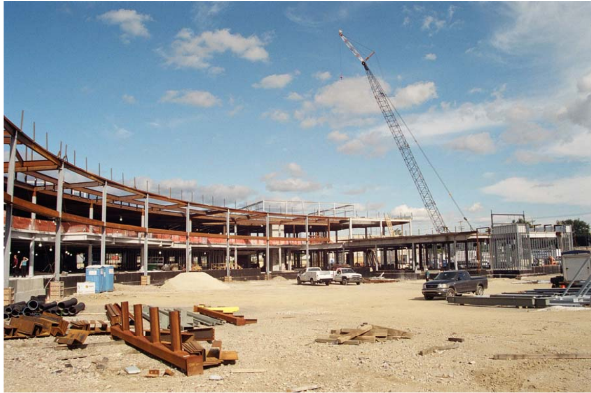
View of steel framing at the south façade.
