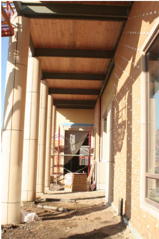
View of exposed steel and wood decking at the east porch.
