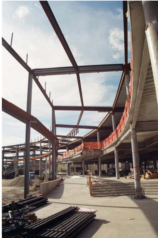
View of steel framing at two story main lobby.
